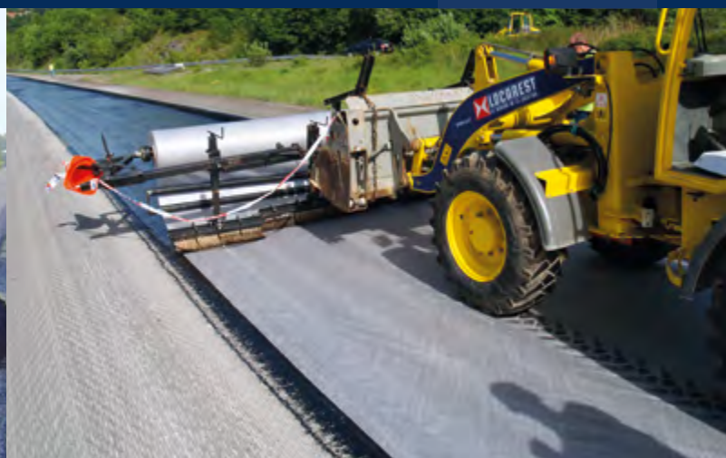
Maintenance of an old asphalt road with regulating layer
